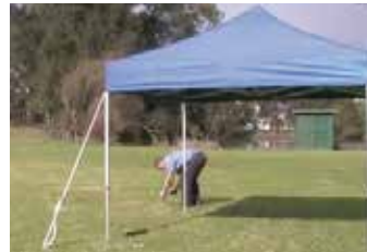
11. Secure with pegs and guy-ropes if it is windy.
